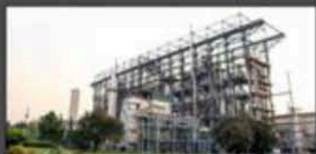
Heavy Water Plant, Hazira, Gujarat (Heavy Water)
