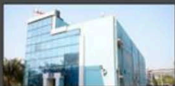
Heavy Water Board Facility Mumbai, Maharashtra (Co, Ni, H 2 , etc.)
