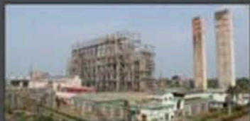
Heavy Water Plant Thal, Maharashtra (Heavy Water)
