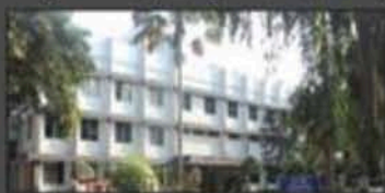
Heavy Water Board Facility Vadodara, Gujarat (Nuclear solvents, Sodium Metal Potassium metal, D 2 Gas)
