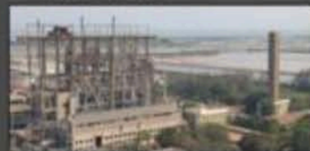
Heavy Water Plant, Tuticorin, Tamil Nadu (Heavy Water, Nuclear solvents, Rare Material)
