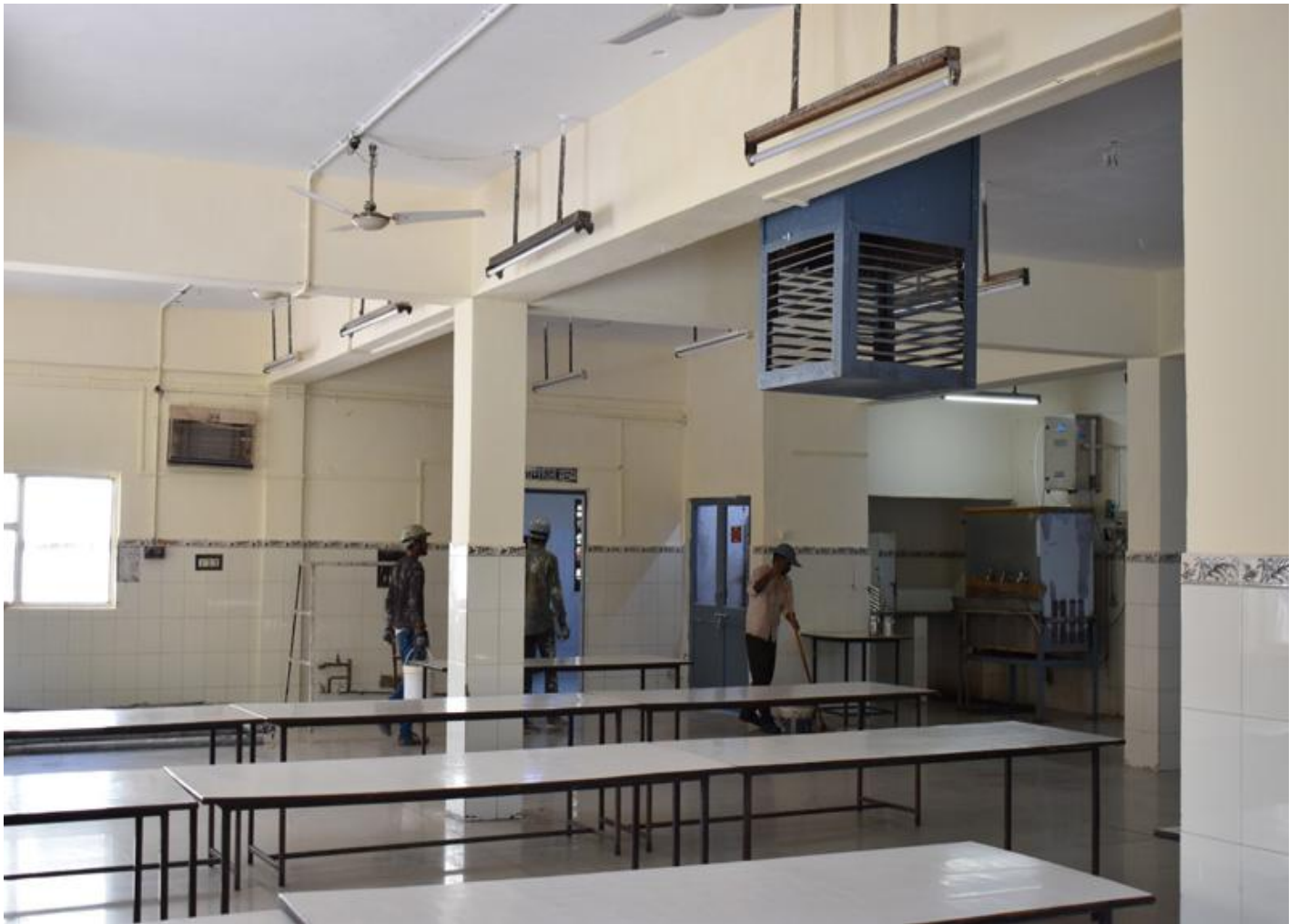
19/2/2025 to 21/2/2025 – Painting and makeover activities at HWP(K) site Canteen
