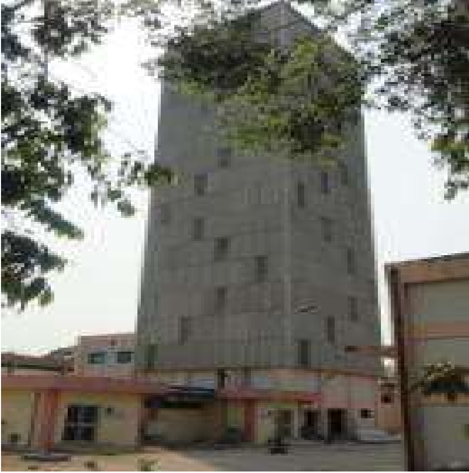
O-18 Water Production Facility
